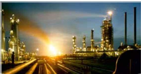
SOCAR STAR REFINERY - TURKEY
