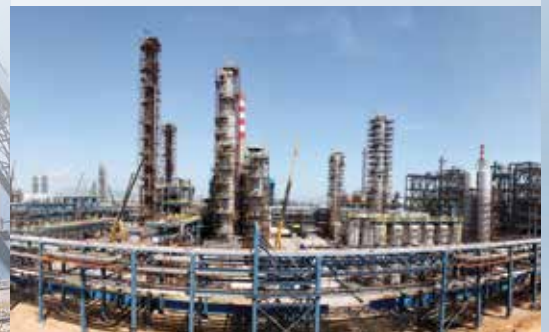
Power Generation Industry
