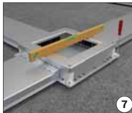
7 Level the junction box using a spirit level.
