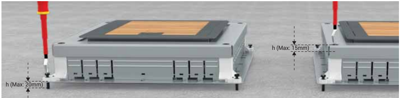
Before Screed Height Adjustment (20mm)
