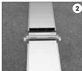
2 Connect the conduits together.
