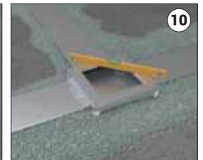
10 Level the connection using a spirit level. Complete the system connections.
