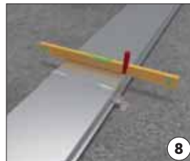
8 Level the connection using a water gauge.
